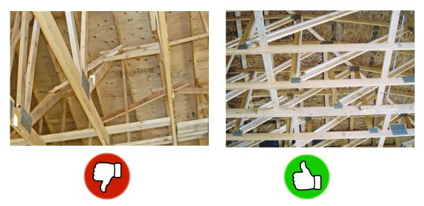
It is the Truss Designers duty to review the truss web configurations to ensure that if there is a situation where at least 3 truss configurations do not align to switch the bracing from CLB to T-Bracing.
